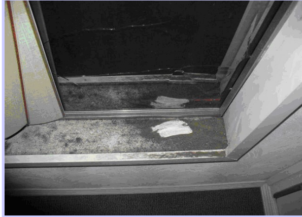
Settled char particulates on windowsill from structural fire in close proximity.
