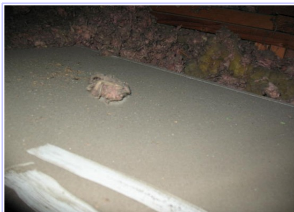
Settled particulates on reverse side of access panel and insulation in the attic.
