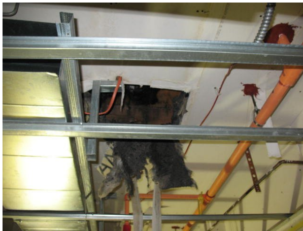
Soot and Char in Ceiling Areas
