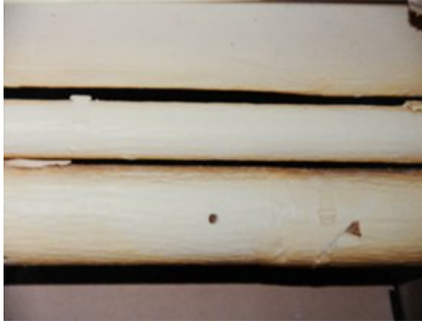
Shot of Aircell Asbestos
