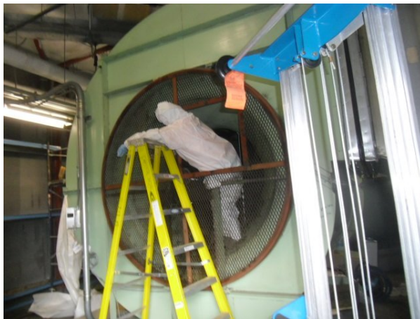
Mechanical Room Air Supply Fan Maintenance
