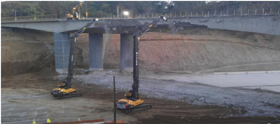
Bridge Demolition over the 405 Freeway on July 16, 2011
